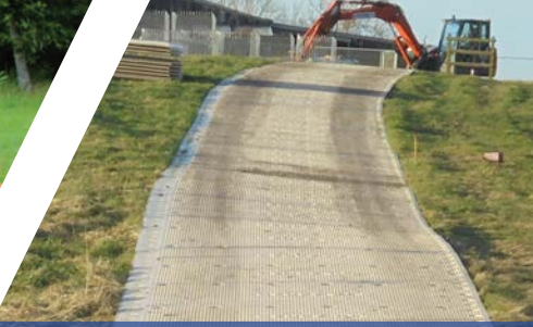
Heavy-haul Temporary Roadways and Accessways
